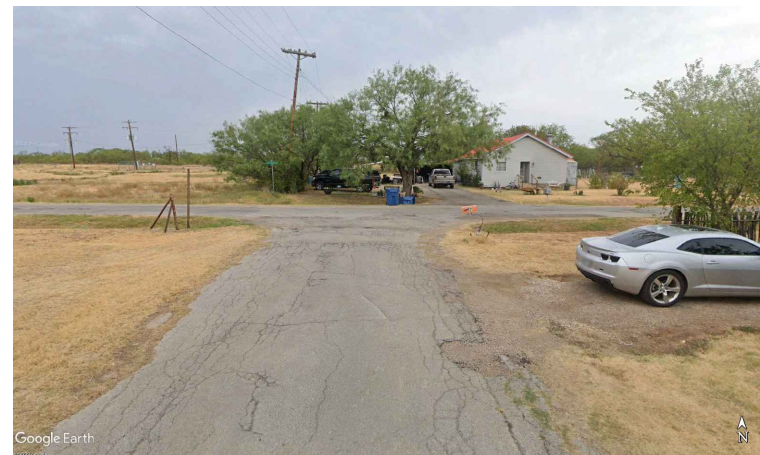
FIFTH ST INTERSECTION
