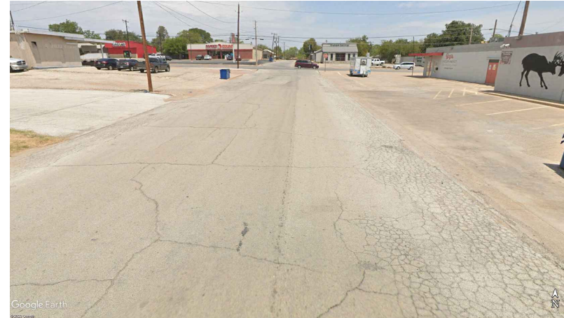
WALKER ST INTERSECTION
