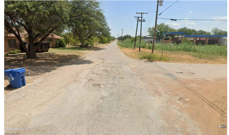
OAKWOOD ST INTERSECTION
