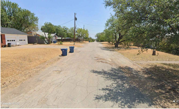
WILSON ST INTERSECTION
