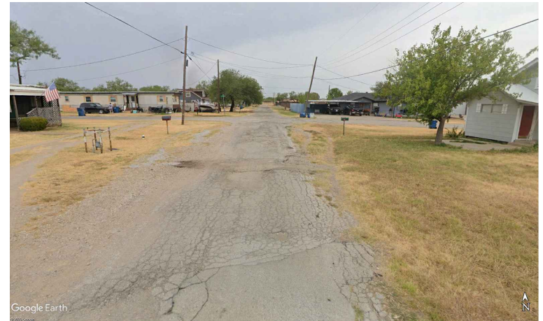
WALL ST INTERSECTION
