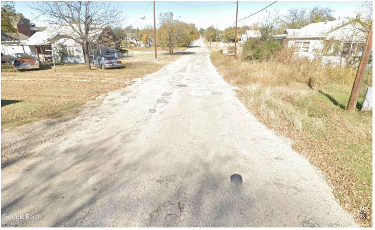
WALKER ST INTERSECTION
