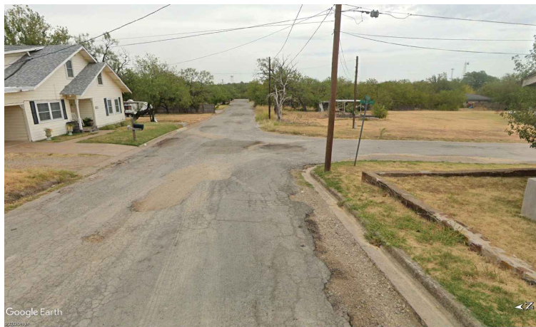
MCAMIS ST INTERSECTION
