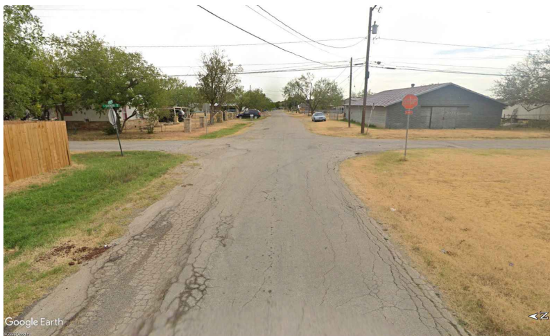
OAKWOOD ST INTERSECTION
