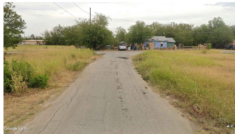
COURT ST INTERSECTION
