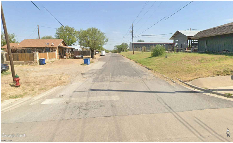
WALKER ST INTERSECTION
