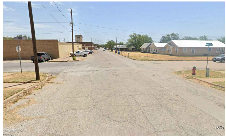
MCAMIS ST INTERSECTION
