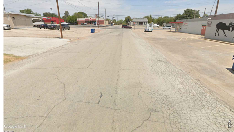
WALKER ST INTERSECTION
